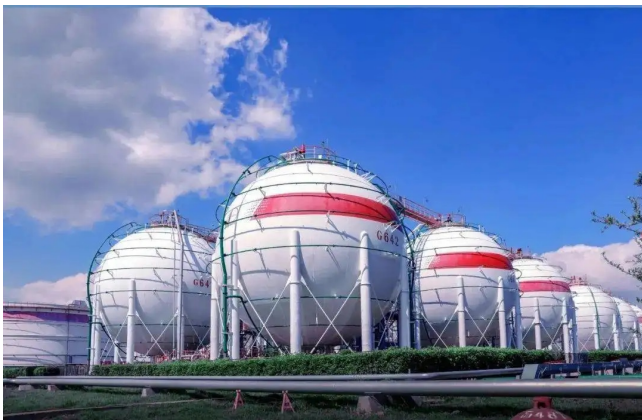
oil depot and chemical tank area
