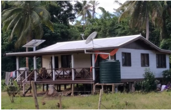
home solar photovoltaic power generation emergency system
