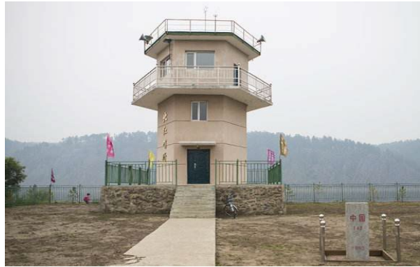
solar PV power generation emergency system in remote and power shortage places
